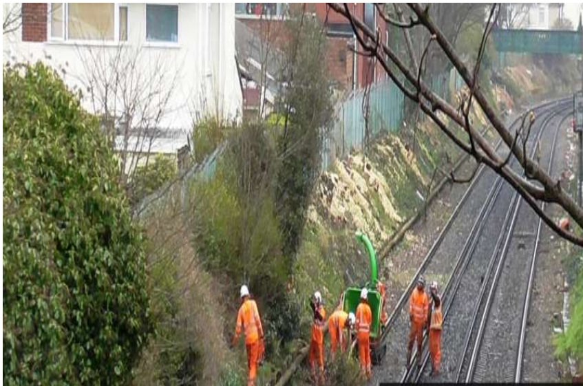
Clearance of trees on track embankment
